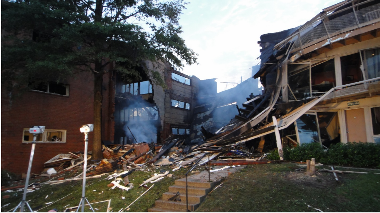
Figure 2. Buildings 8701 (right-center) and 8703 (left) Arliss Street, Silver Spring, Maryland, after the explosion and fire. (Photograph provided by the Public Service Commission of Maryland.)
